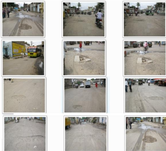
Fig. 9. Sample database for pot holes
