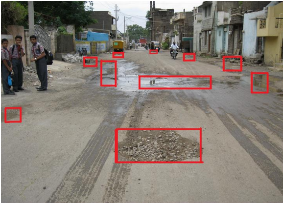
Fig. 13. Sample result of pot hole detection
