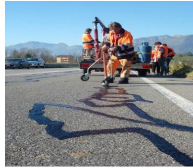
Fig. 3. SEALMASS M5 sealing equipment.
