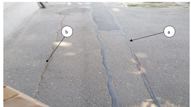
Fig. 11. Cracks in asphalt: a – repair of the crack classic method, b - crack affected by weather
