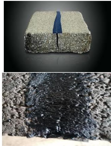
Fig. 10. Cracks sealing by friction method
