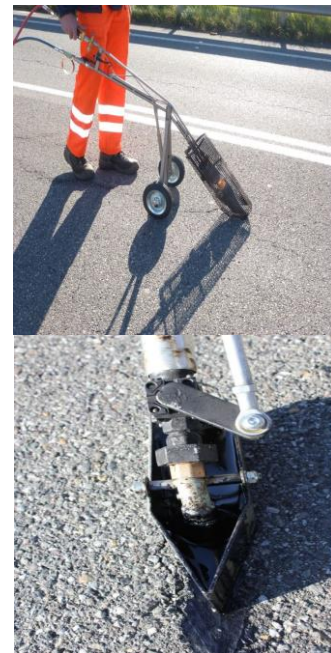
Fig. 4. Liquid bitumen application device.
