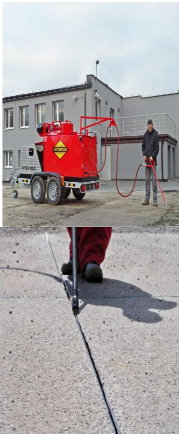
Fig. 6. Device for bitumen application into the crack.
